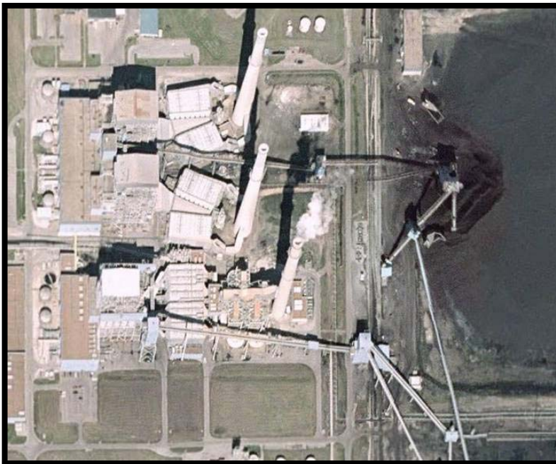
Fayette Power Project, Units 1, 2 and 3 Texas
